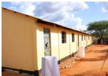
The new block that was completed in April 2019
