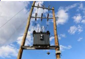
Electricity connection to the area was courtesy of the school. This Transformer stands in the school compound
